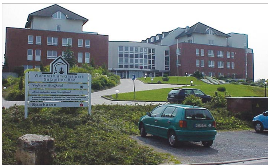
Figure 9. Today the Chemischen Fabrik of Unger's Erban & Company is gone and is replaced by a “Wohnstift”—an old folks’ home on Kurpark am Greif (“Healthpark of the Griffin”) (N52° 02.38 E10° 22.65).
